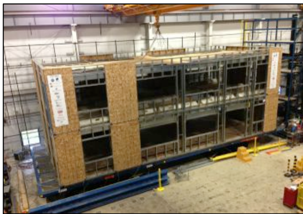
(a) Phase 1 completed building
