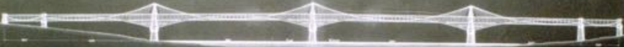
ST. LOUIS BRIDGE. 1873
