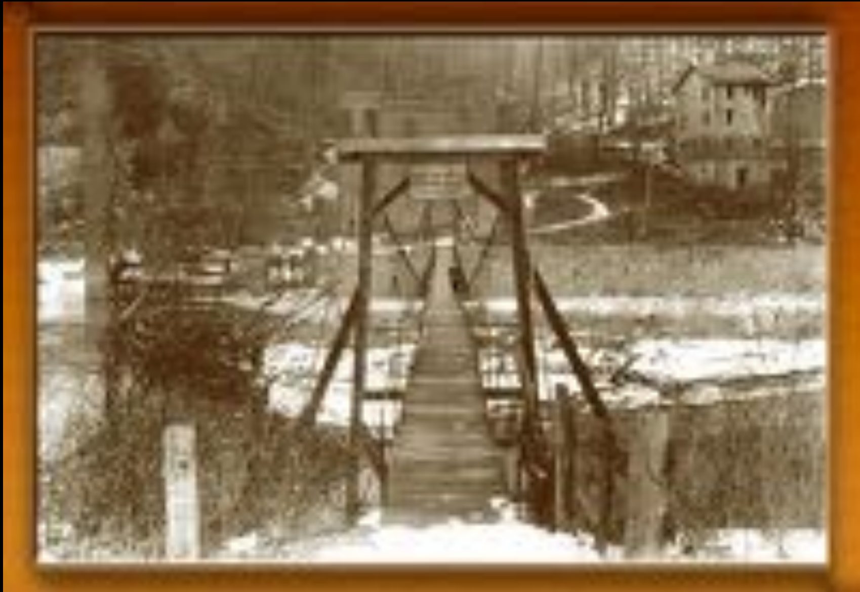
Local unstiffened suspension bridge example Patapsco Valley State Park “Swinging Bridge” (Early 1800’s)
