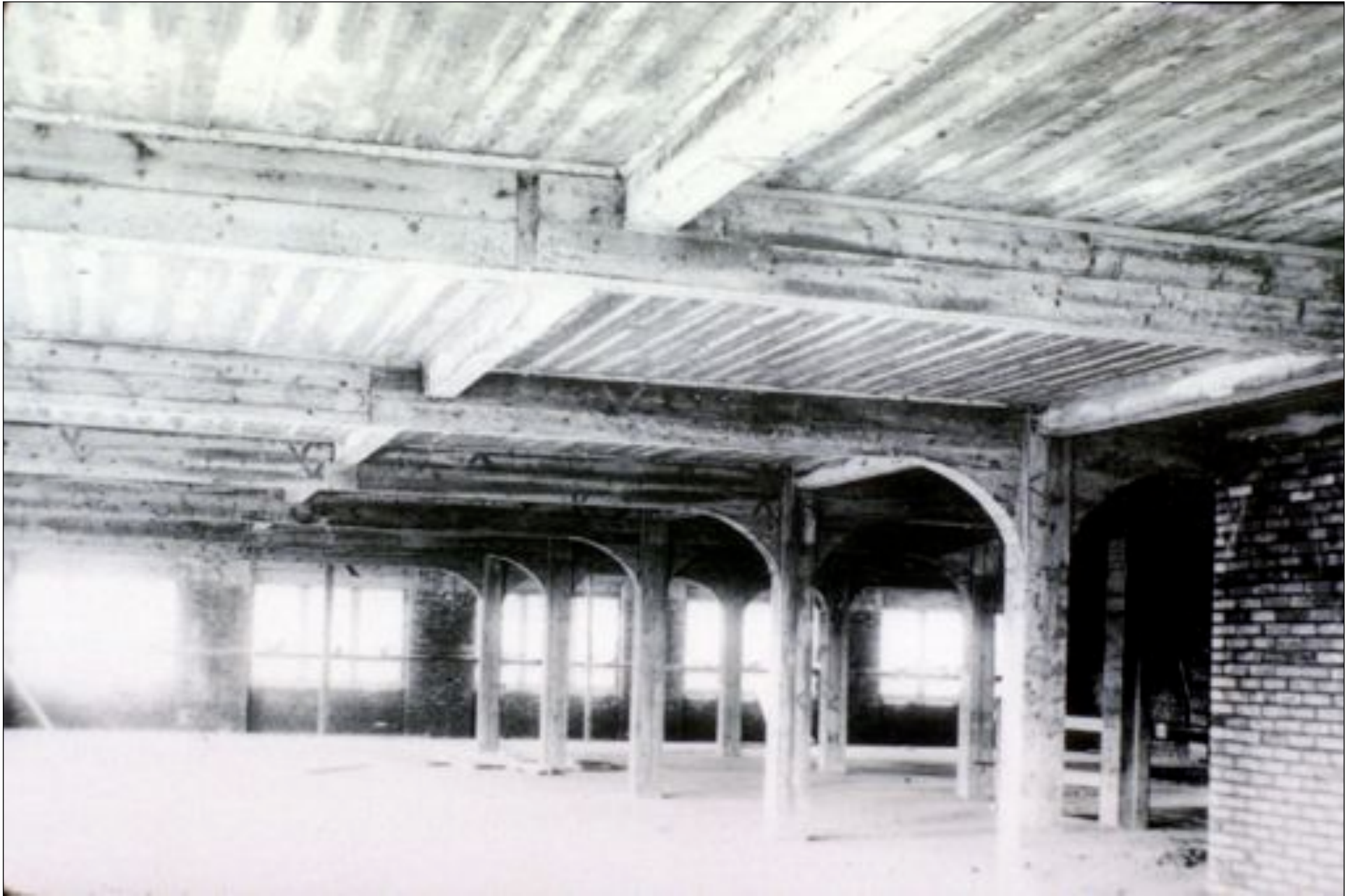
St. Gallen Warehouse (1908) Robert Maillart
