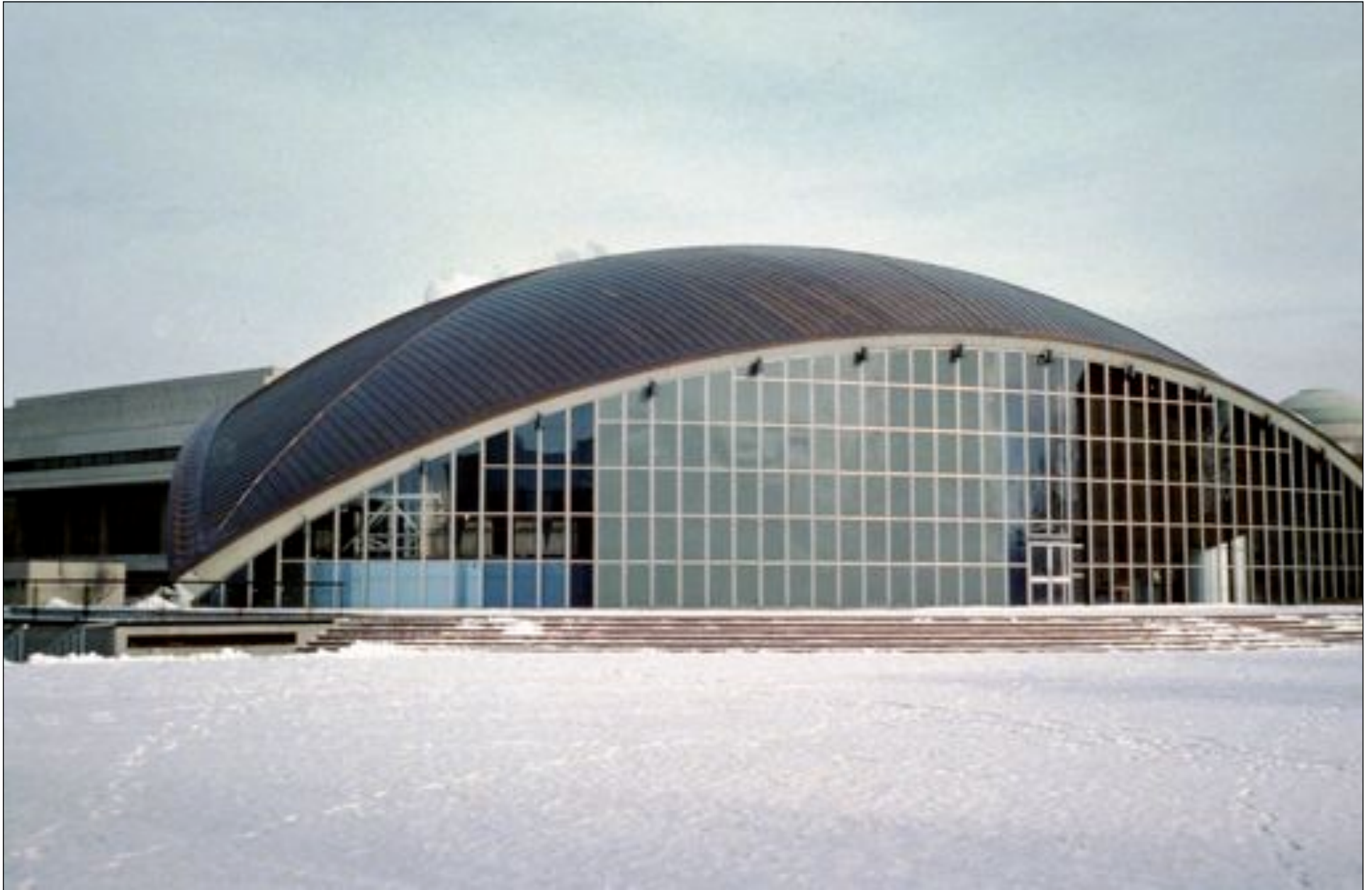
Kresge Auditorium (1955) Eero Saarinen, architect
