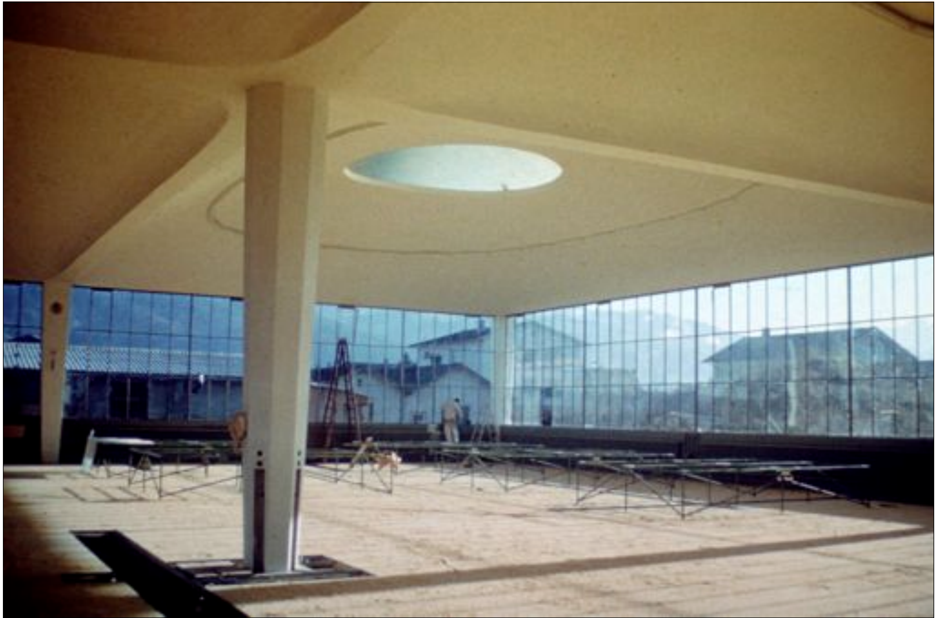
Eschmann Company Building (1958) Heinz Isler
