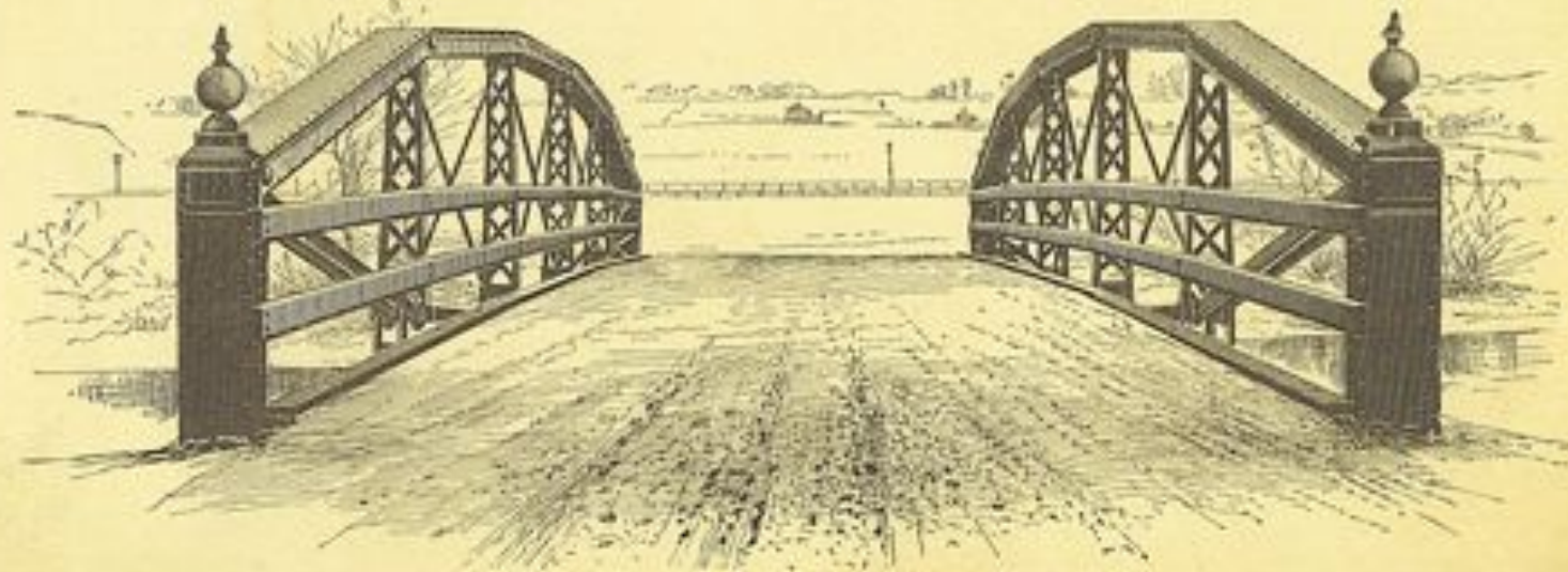
BRIDGE AT JAMESTOWN, CHAUTAUQUA COUNTY, N. Y. Span, 70 feet. Roadway, 10 feet wide.
