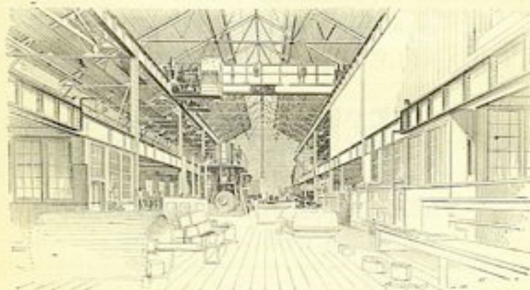
The above illustration is taken direct from a photograph and shows the interior of a Forge Shop designed and built by us for Wm. Cramp & Sons Ship and Engine Building Co., at Philadelphia, Pa. The Forge Shop is 59 ft. in width and 50 ft. in length, the adjacent Boiler Shop (shown on the right) being 45 ft. in width and 350 ft. in length. The Smith Shop is controlled by a Travelling Crane as shown. The building is covered with Corrugated Iron.
