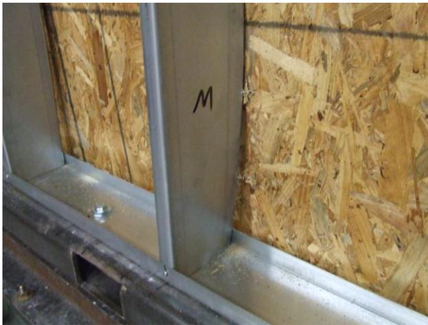
Missing fasteners at the bottom
