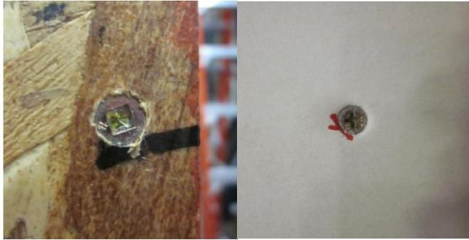
Figure 11 Appropriate fastening in OSB and gypsum board
