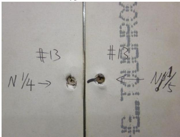
Vertical seam fasteners
