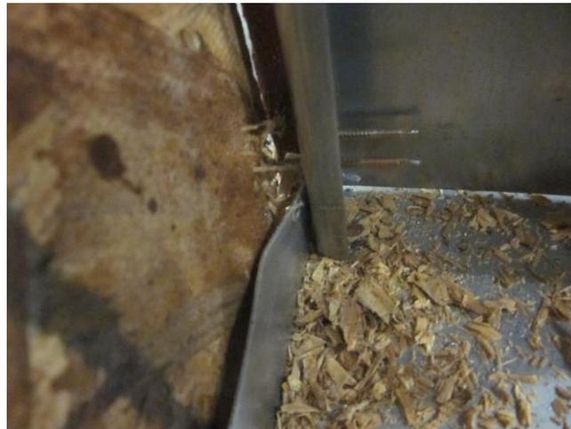
Additional stud at vertical seam (Bottom)
