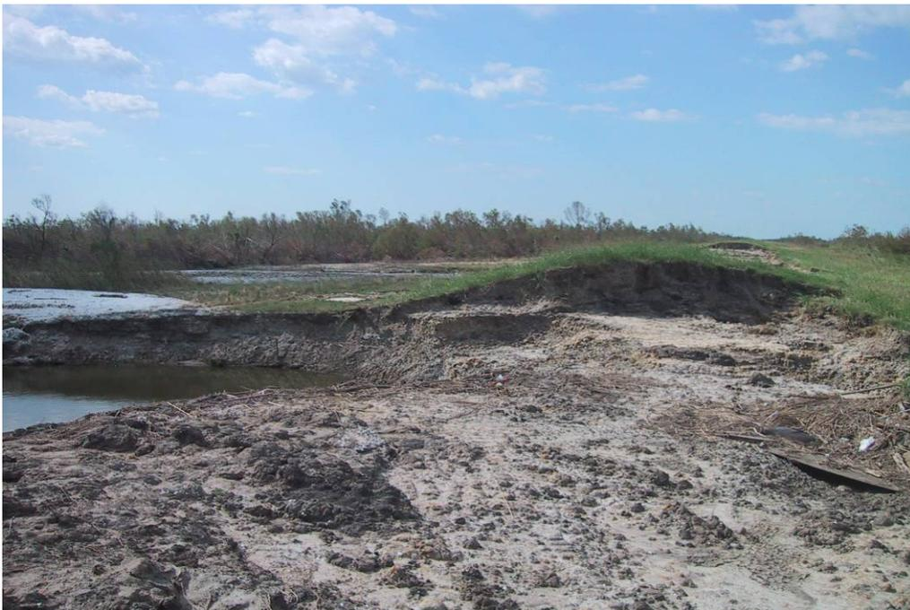
Figure 4.24: Failure of earth levee on southwest bank of MRGO adjacent to the Bayou Dupree gate (L. Wooten, October 6, 2005).
