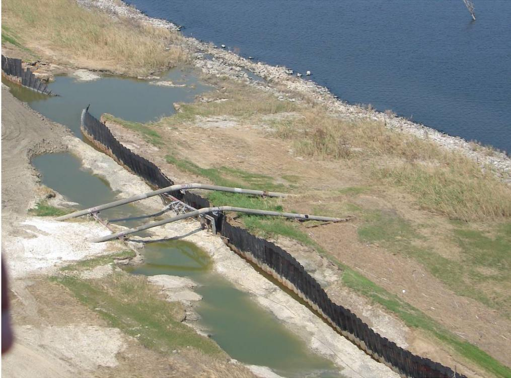
Figure 4.21: Levee failure on southwestern bank of MRGO between Bayou Bienvenue (where barge is aground on I-wall) and Bayou Dupree. Note severe erosion and scouring (L. Harder, October 14, 2005).
