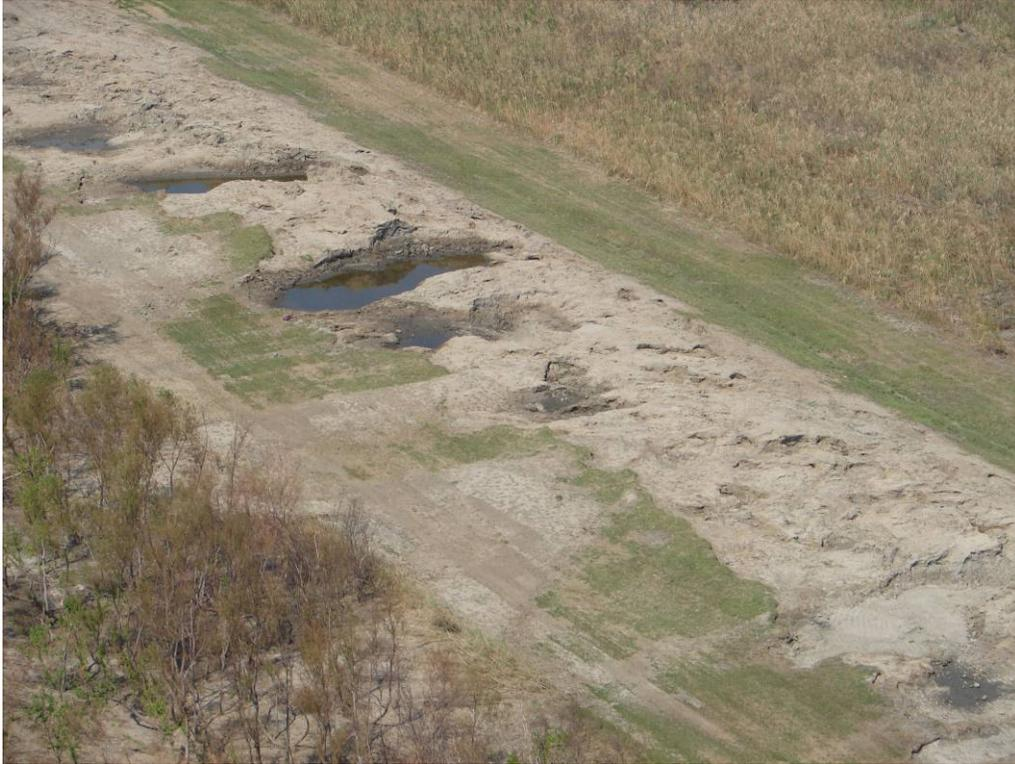
Figure 4.25: Overtopping obliterated earth levee along southwestern bank of MRGO, within two miles southeast of Bayou Dupree. Note deep scour at the levee foundation level (L. Harder, October 14, 2005).
