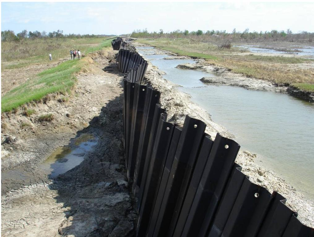
Figure 4.20: Failure of earth levee with steel sheetpile barrier on the southeast bank of the MRGO. Note severe erosion and scour (L. Wooten, October 6, 2005).
