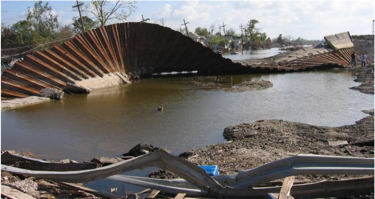
Figure 4.10: Overturned I-wall system at north breach of Lower Ninth Ward (J. Wartman, October 4, 2005).
