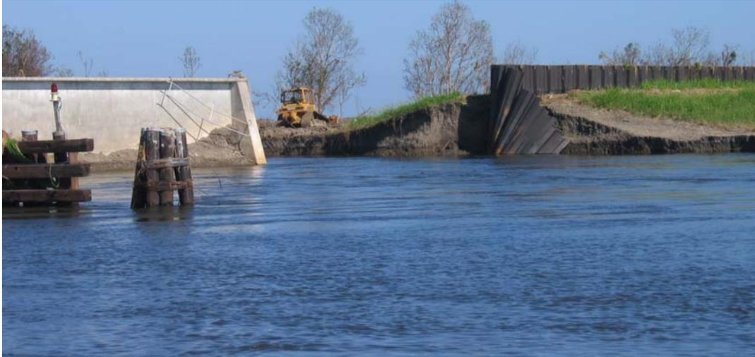
Figure 4.13: Sheet pile breach at the Bayou Bienvenue Gate (J. Wartman, October 5, 2005).
