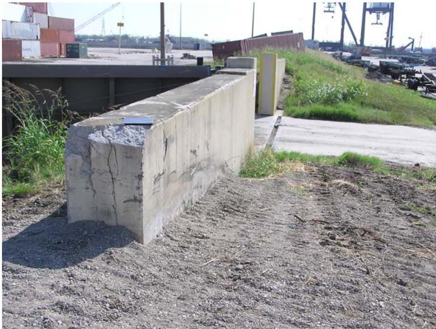
Figure 2.32: Common structural wall (with flood gate) and earthen levee transition problem with erosion at the contact between the earth and concrete sections.
