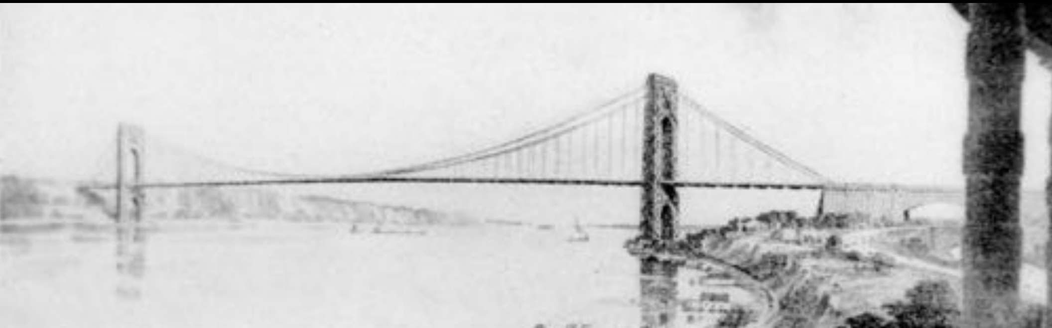
George Washington Bridge - Othmar Ammann - 3500 ft [1067 m] - 1931
