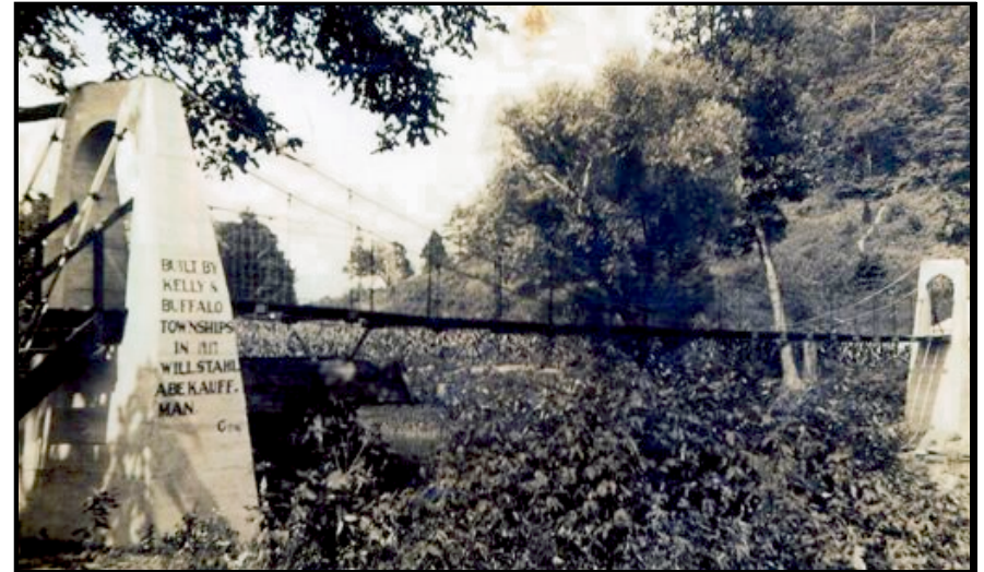
Buffalo Creek Bridge (1917)
